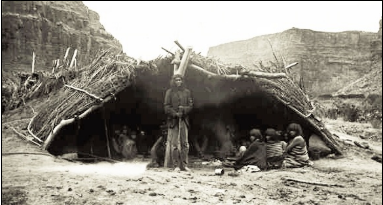
Plate 6.3-8. Three-sided lean-to structure characterized as a “double lean-to” that was utilized at Havasupai and depicted in the Handbook of North American Indians, Southwest, Vol. II (Schwartz 1983, Figure 42).
