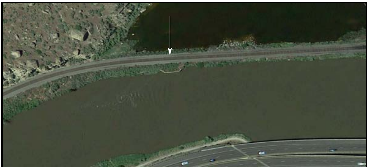
Plate 3. Google Earth image of the likely location of a remaining dam abutment.
