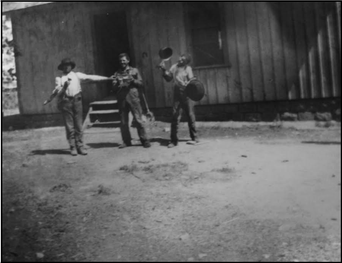
Plate 7. “Unknown section men clown around outside Tunnel section house in 1907” (Mangnall 2015). Note the formed blocks used in the foundation. None were found on the site.
