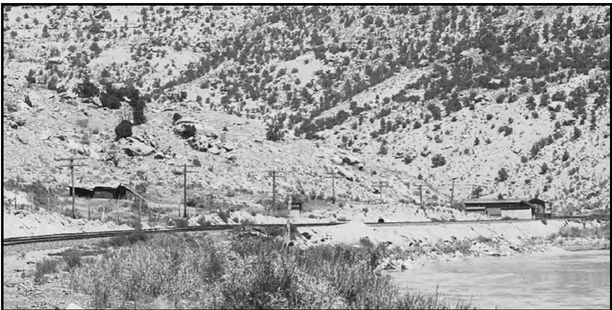
Plate 4. Close-up view of structures associated with Tunnel Siding and Station (Denver Public Library, Western History Collection [Call number GB-6485]).
