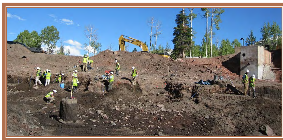
Plate 2. ZRFS excavation near spillway Summer of 2011.
